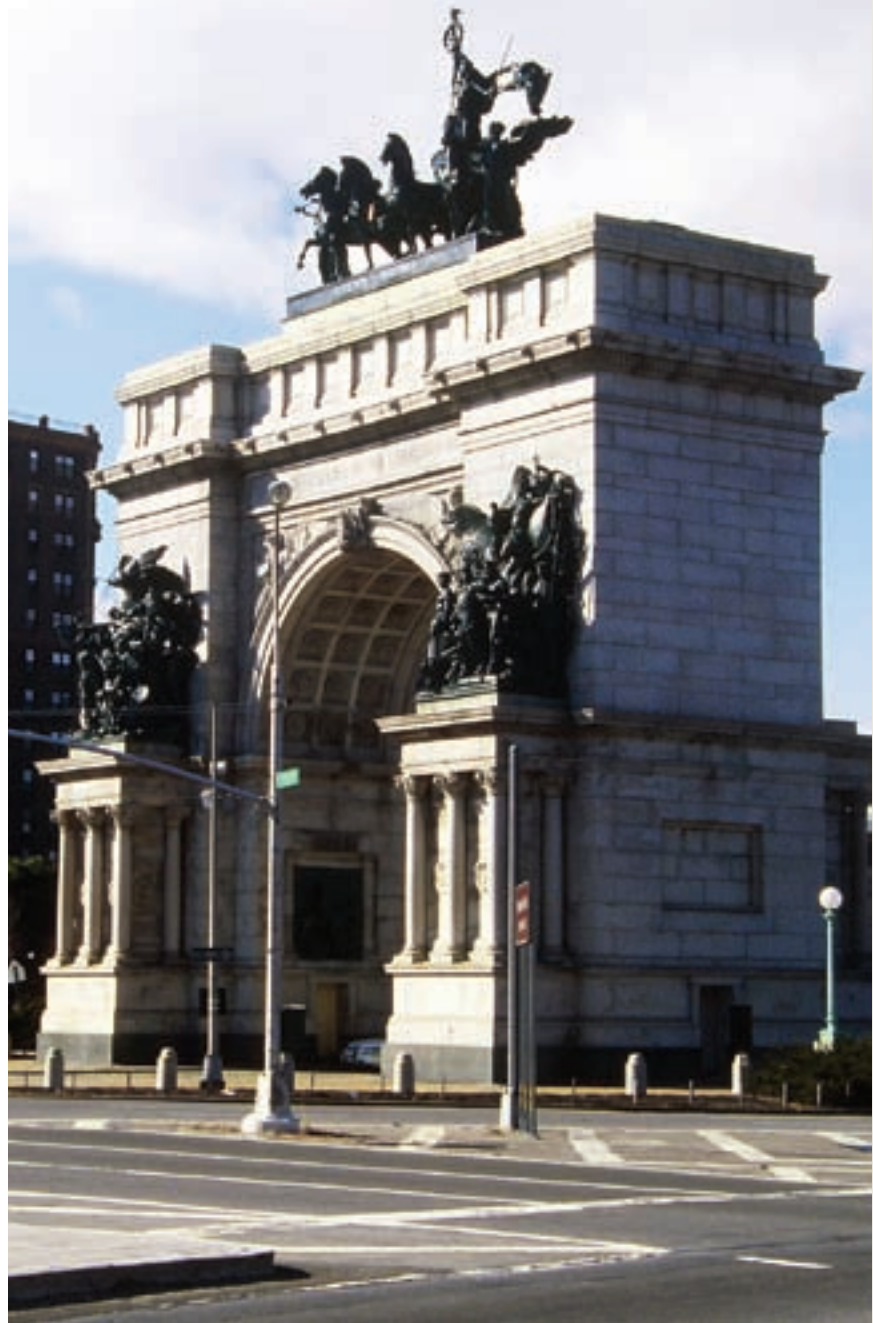
The Memorial Arch at Grand Army Plaza
